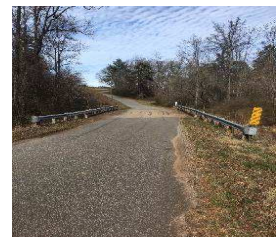
Blackwell Rd bridge
