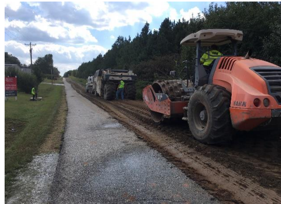
Brookshire Road Repair
