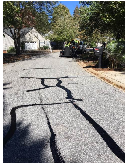
Crack Sealing in Riverside Chase
