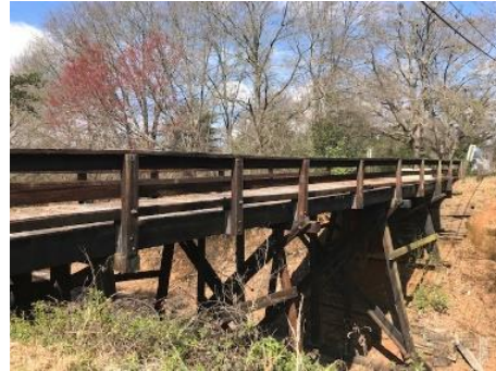
CSX RR Bridge at Biblebrook
