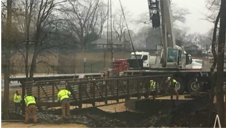
Century Park Pedestrian Bridge Installation
